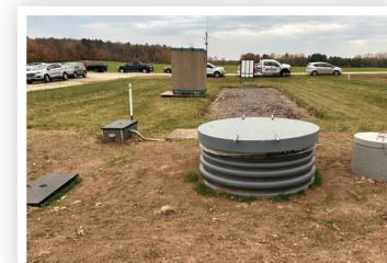
A view looking west of the Phosphorus Removal System and Denitrifying Bioreactor. Components include water control structures, HDPE access manhole to monitor flow, concrete holding tank riser, diversion embankment, woodchip bioreactor, and USGS monitoring controls structure. Photo credit: Whitney Prestby, UW-Madison Division of Extension
